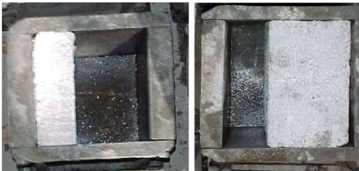
a) Styrofoam to form block-out
